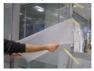
Finally remove the 8150 film from the glass.
